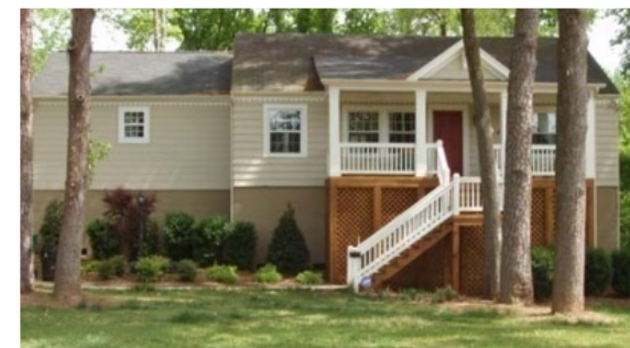
Structure elevations and floodproofing
